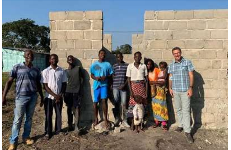
House under construction to be donated to Chico and Lucia, who will live there with four of their seven children.
